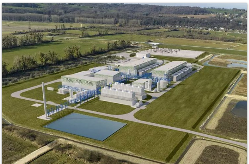
Normand'Hy Electrolyzer plant under development in France
